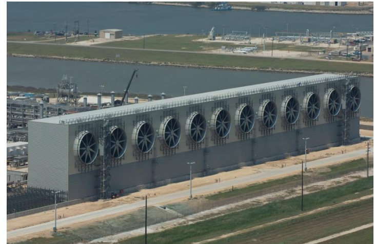
Picture: VE-Tower June. 2008. Courtesy of Freeport LNG
